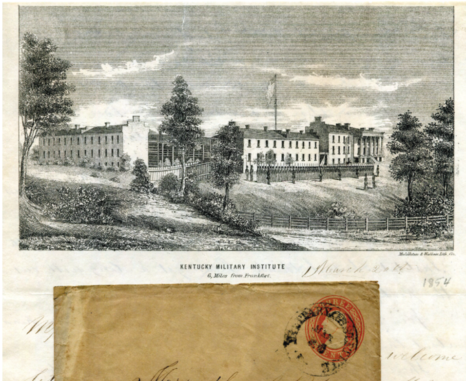
Figure 2. Illustrated lettersheet depicting the Kentucky Military Institute in 1853-54. The cadets are seen in formation on the parade ground. Part of the 3¢ entire envelope that carried this letter, cancelled with the Type 1 marking, is also shown.
